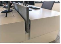
The architects used felt—produced from recycled PET bottles—in wall finishes and desk panels for the purpose sound absorption. (photo: Christiaan de Bruijne)
